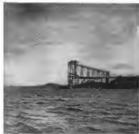
... completed it will be one nd in the world. Engineers of progress the job will be Philip J. Corbett.)
